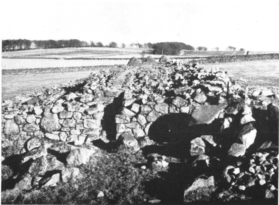
PLATE 42 Kingswells consumption dyke, \frac{1}{4} mile long, 20 feet wide and 6-8 feet high.
